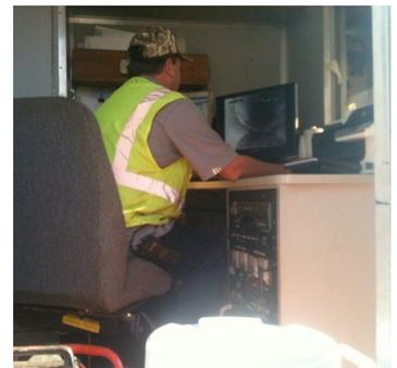
**PHOTO 6F.** ACC Stormwater worker uses a camera to find the exact location and extent of the two damaged sewage pipes.
