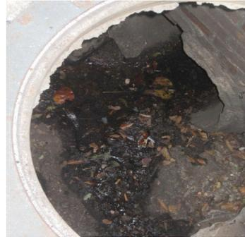
**PHOTO 6B.** Flow in dry weather in a stormwater pipe suggests sewage leak.
