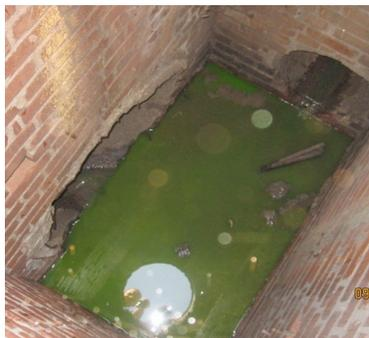
**PHOTO 6D.** Green dye is flushed down the toilet of a nearby business, helping hone exact location of leak.
