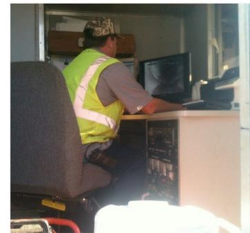
**PHOTO 6F.** ACC Stormwater worker uses a camera to find the exact location and extent of the two damaged sewage pipes.
