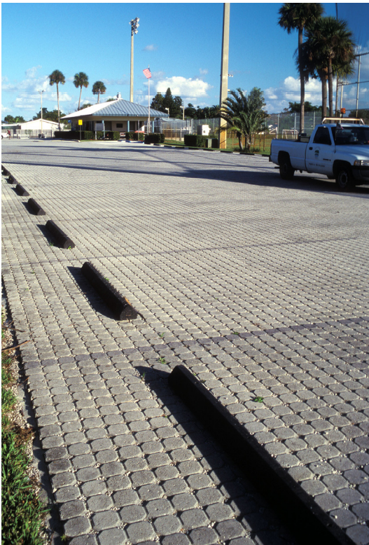
Three examples of modular pavers. Photos by Bruce K. Ferguson.
