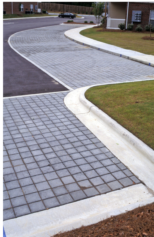
Three examples of modular pavers. Photos by Bruce K. Ferguson.
