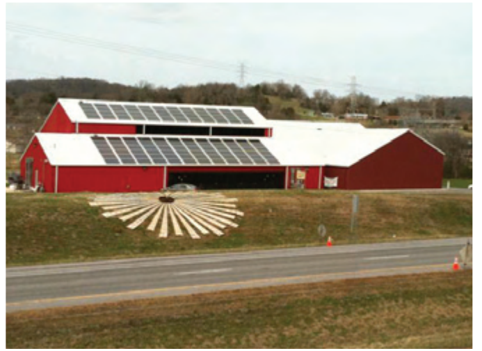
Art Center of Cannon County, - Woodbury, TN. Photo credit LightWave Solar.
