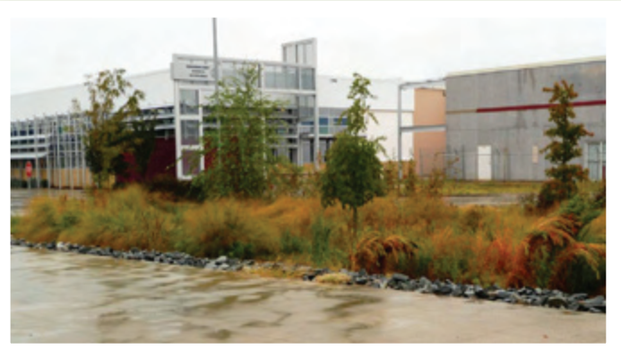
Valarie C. Woodward Center received LEED Silver certification. Outdoor activities included bioretention areas to reduce runoff and allow for greater filtration of stormwater.
