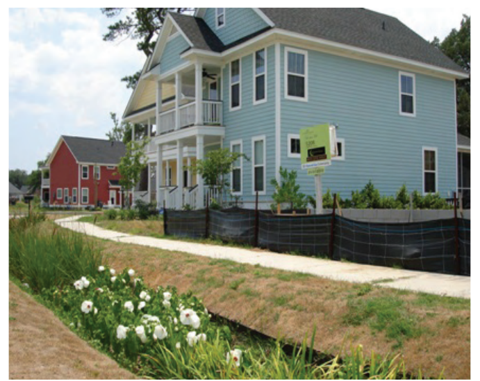
Bioswales enhance water infiltration into the soil, reducing runoff. Photo credits Southeast Watershed Forum.
