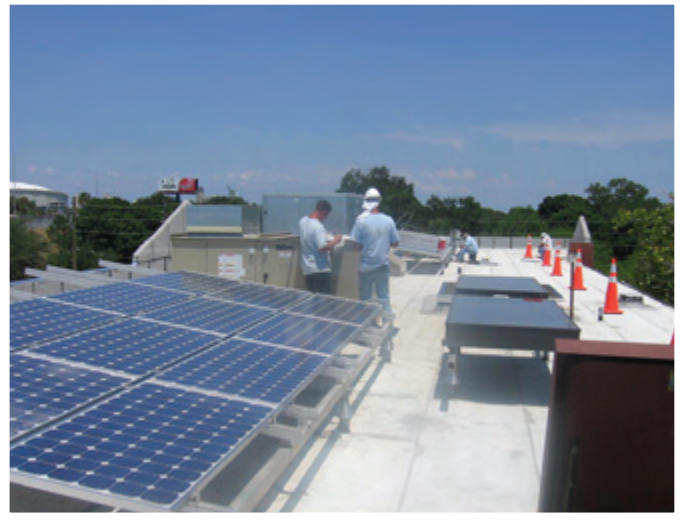
Solar water heater and panels. St. Petersburg, Florida.
