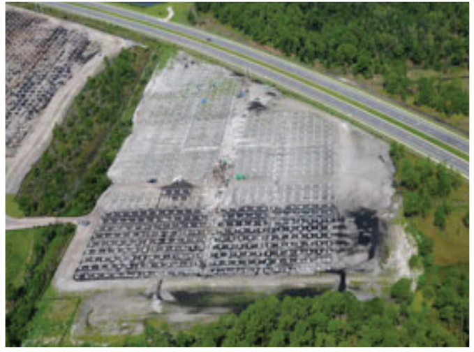
The first solar farm in Orange County at OUC’s Curtis H. Stanton Energy Center. The 5.9-Megawatt solar photovoltaic (PV) can generate enough renewable energy to power more than 600 homes.
