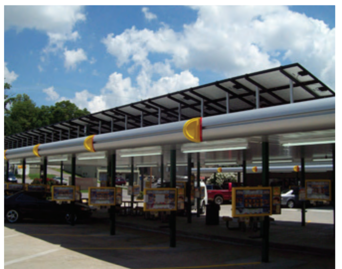
Solar power supports this Sonic Drive-In in Nashville. Photo credit LightWave Solar.
