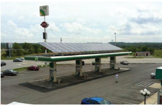
Solar powered truck stop in Crossville, TN. Photo credit LightWave Solar.
