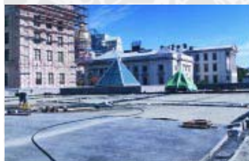
Preparation for the Enkadrain layer at the New Jersey State House.
