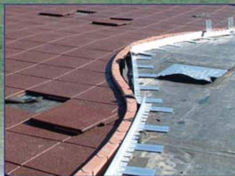
EcoEdge with custom footings prior to install.
