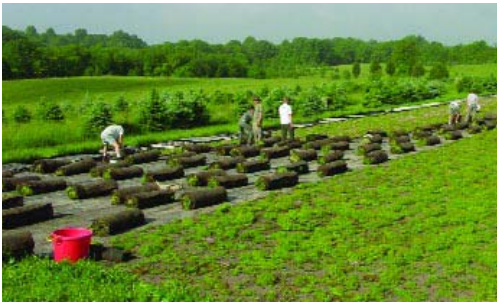
Plants are grown directly in Enkarooft VM and transported to the site ready to unroll.**
